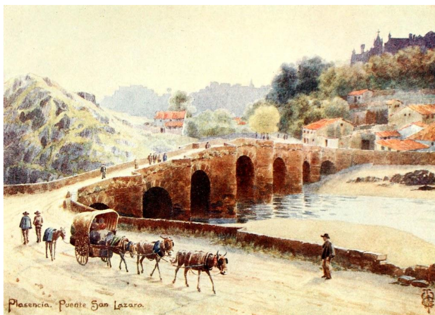
Plasencia. Puente San Lázaro, Edward Wigram (Northern Spain, 1906
